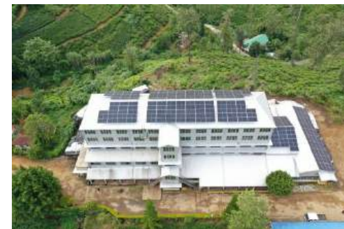
Rooftop Solar Generation
